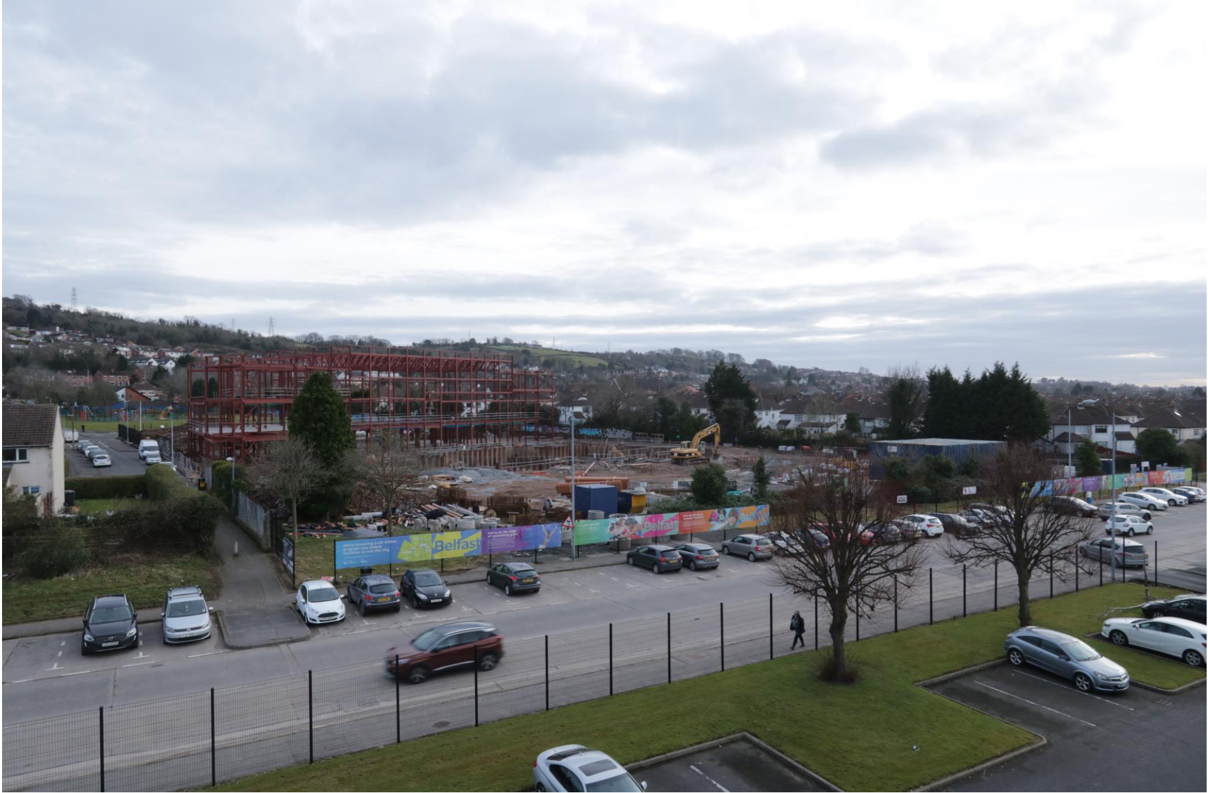
Robinson – Works Underway – March 2018
