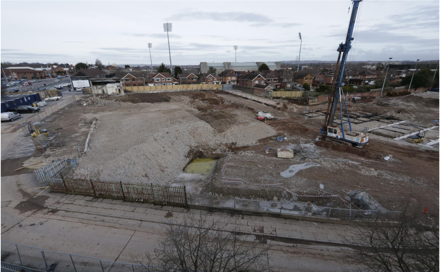
Andersonstown – Works Underway – March 2018
